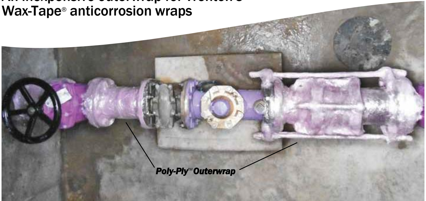
The photo above shows Poly-Ply™ Outerwrap protecting the two sections of pipe covered by Trenton's Wax-Tape® #2 anticorrosion wrap.
